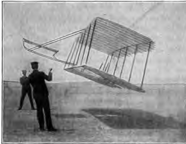
Fig. 5. Flying a Glider as a Kite to Study its Action
